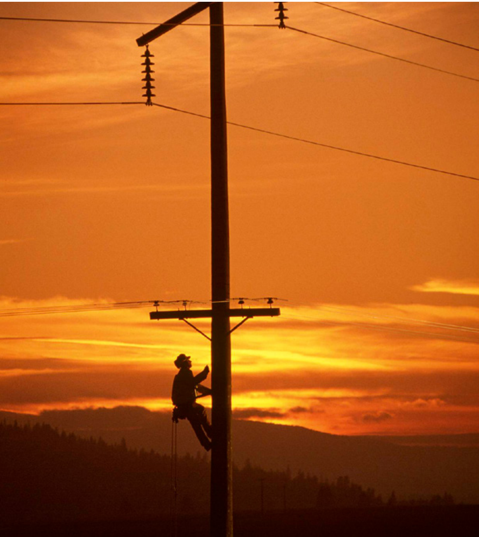
An Avista lineman ascends a utility pole in North Idaho
