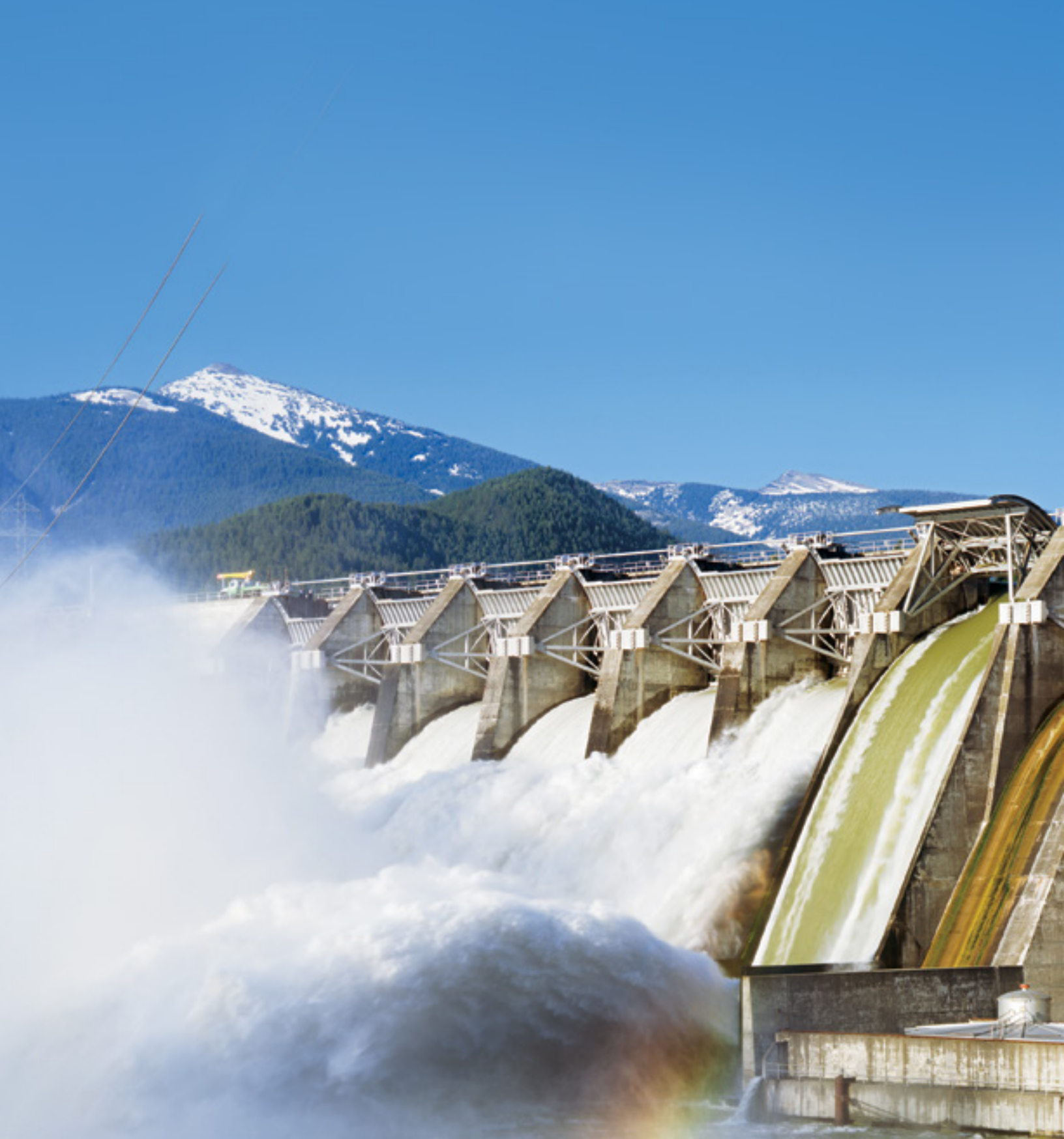
Noxon Rapids Dam, Clark Fork River, northwest Montana
